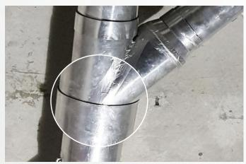
All junctions along longitudinal pipe sections must have adjacent material segments overlapped.
