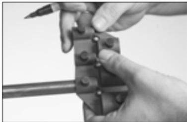
Tectite push fittings – insertion depth for 10 - 28 mm tube (all variants)
