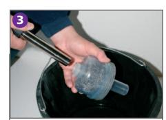
Once removed, place the clear base over a bucket. Unscrew and remove the magnet cap and rinse the sheath.
