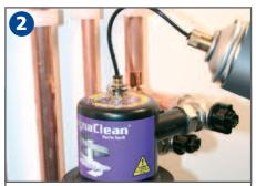
Wait five seconds before removing the adaptor. The Pro-Fill air vent will accept all market-leading chemicals in either liquid or concentrate form.
