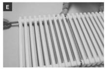
Use the nipple turning key to tighten both nipples alternately. The torque should be 90 +/- 10 Nm. Nipples only tightened on one side will cause leaks!
